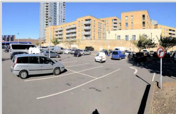
FIGURE 9. - View of The Depot Site from 'B&M' car park (1)
