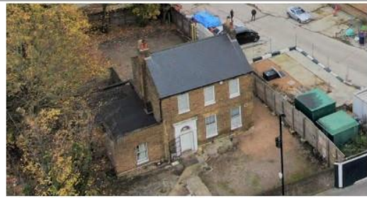
FIGURE 40. - Station Master's House (A)
