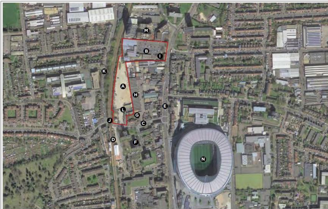
FIGURE 1. - Site Aerial Overview
