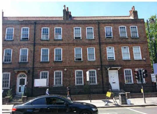
FIGURE 12. - View of the Heritage Block F, Nos. 867-869 High Road (4)
